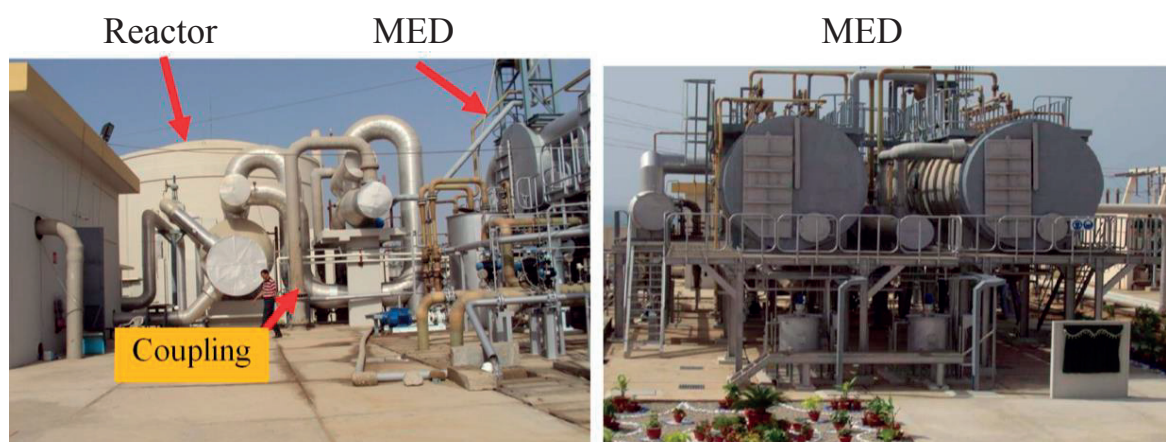
FIG. 19. The KANUPP reactor coupled to the 1600 m 3 /d MED desalination plant.
