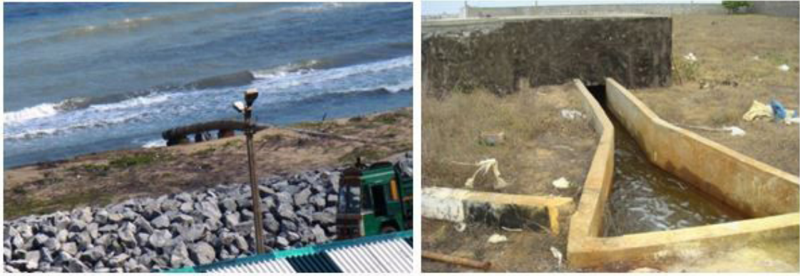
Reject disposal system
